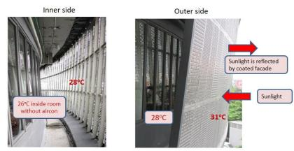
Figure 3. Inner and outer side of double façade system.
